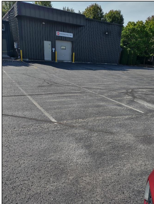
Figure 3: Alternate view of the subject lands
