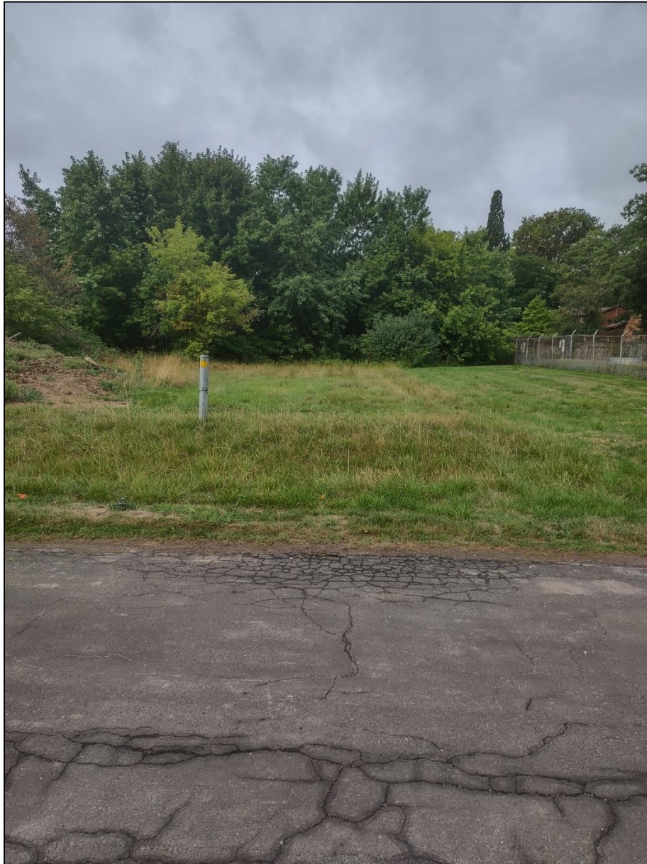
Figure 1: View of Subject Property from Scott Drive
