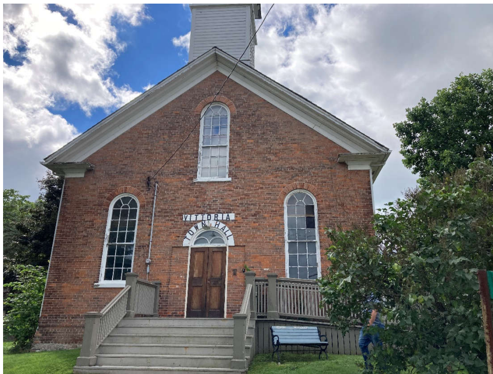
Photo 1: General view of the building
