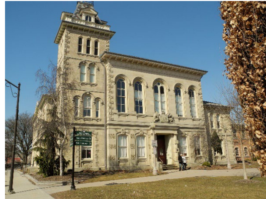
Figure 5: Exterior view of the County Administration Building
