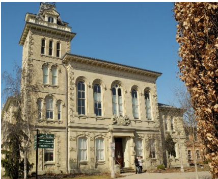
Figure 1: Exterior view of the County Administration Building
