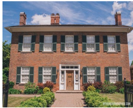
Figure 2: Exterior view of the Norfolk County Archives
