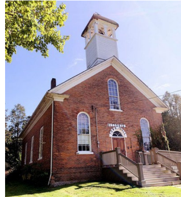
Figure 3: Exterior view of the Vittoria Old Town Hall
