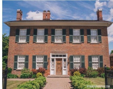
Figure 7: Exterior view of the Norfolk County Archives
