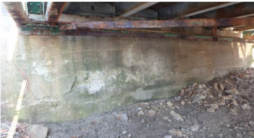
Sever corrosion
